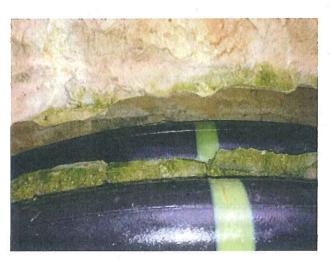
A coarse sandy material was observed entering catch basins through a few of these cracks. Some of the pipe to catch basin connections (CB 30, CB 29 and CB 28) appear to be brick with little or no mortar.
